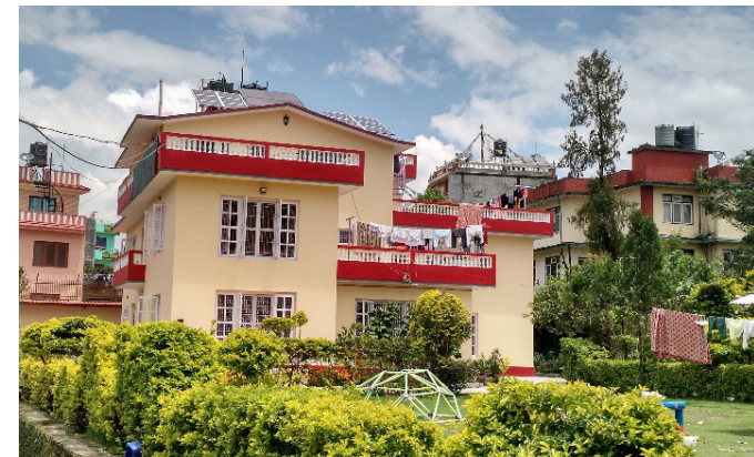
The house underwent extensive reconstruction & retrofitting to withstand any future earthquakes.
